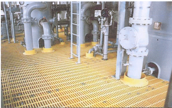
Photograph 1 : Composite Material Gratings on an Offshore Platform
