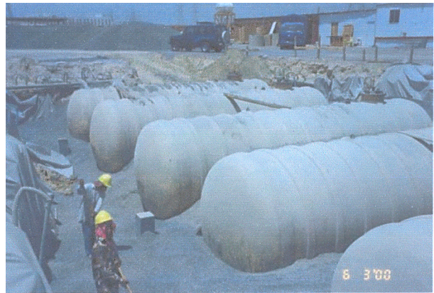
Photograph 4 : Composite Material Underground Tanks Under Installation
