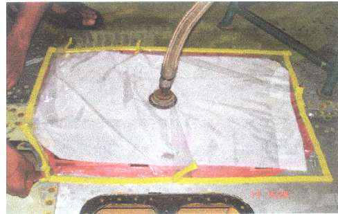
Fig.8 Vacuum Bagging on the Wing Surface
