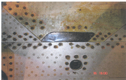
Fig.7 Filler Patch Bonded on the Wing
