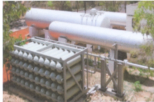
Fig.5 Cascade Assembly and Multi-layered Pressure Vessels
